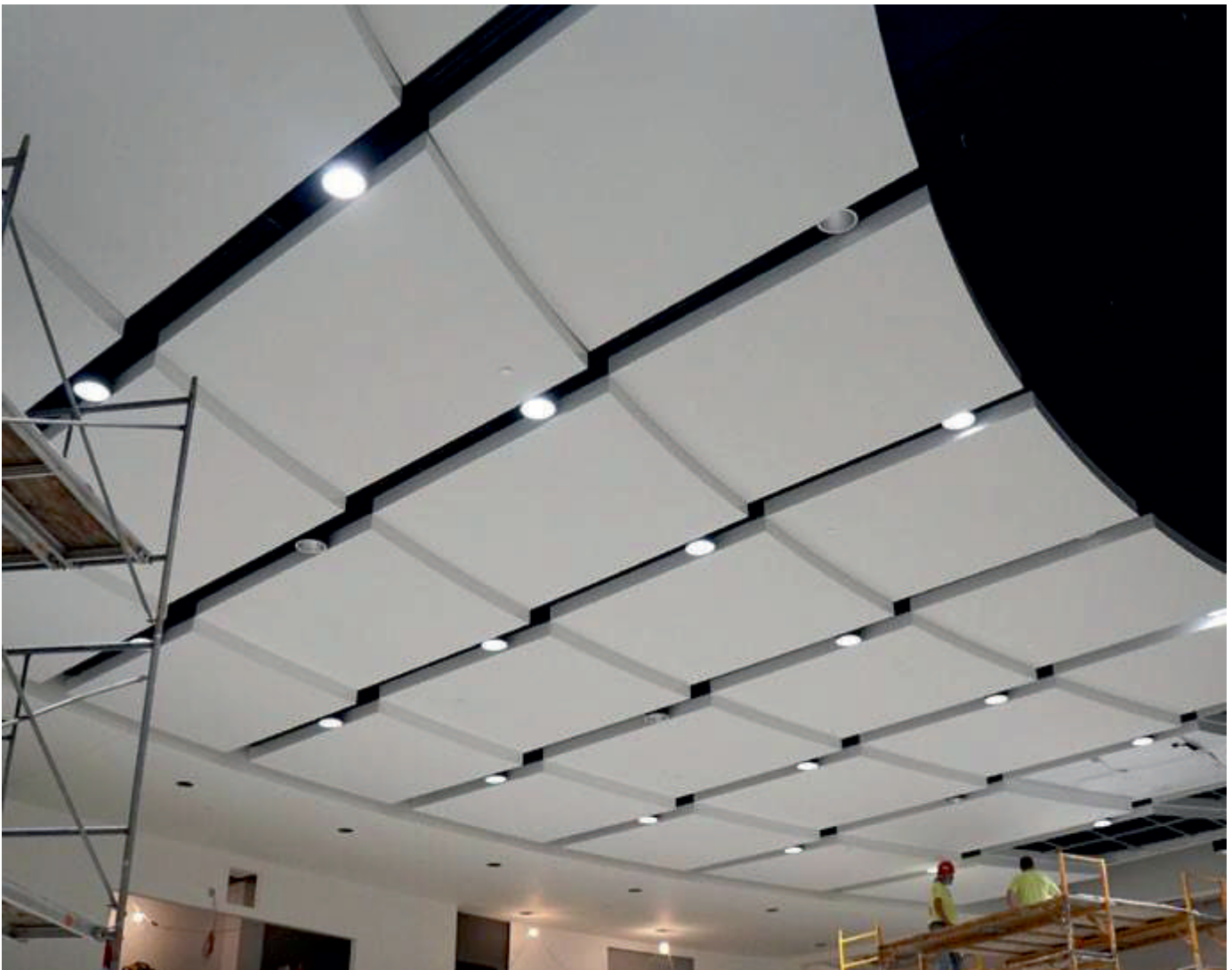
Auditorium Ariel Corporation - USA
